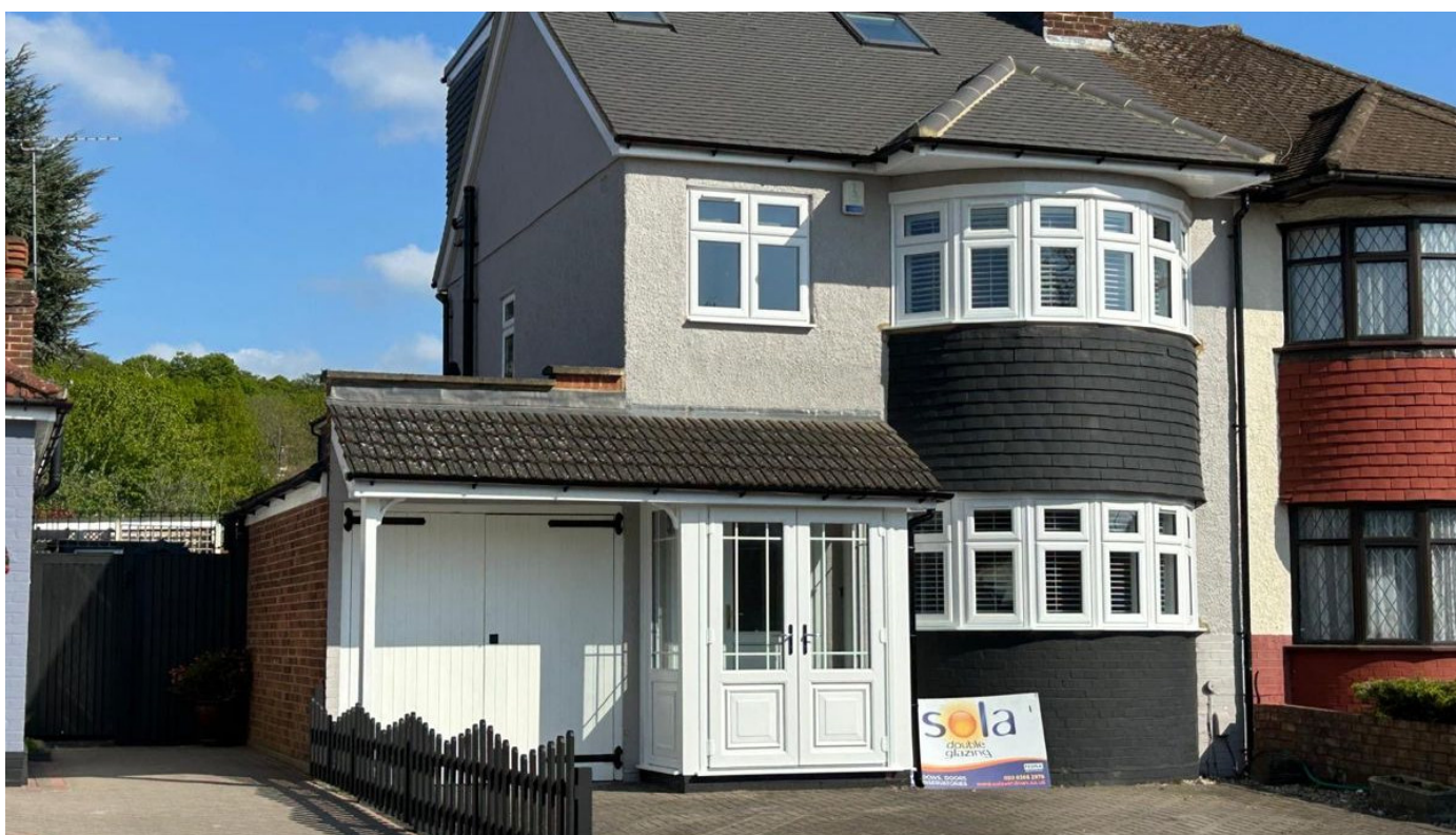
A Sola Windows installation, shown on our website.
